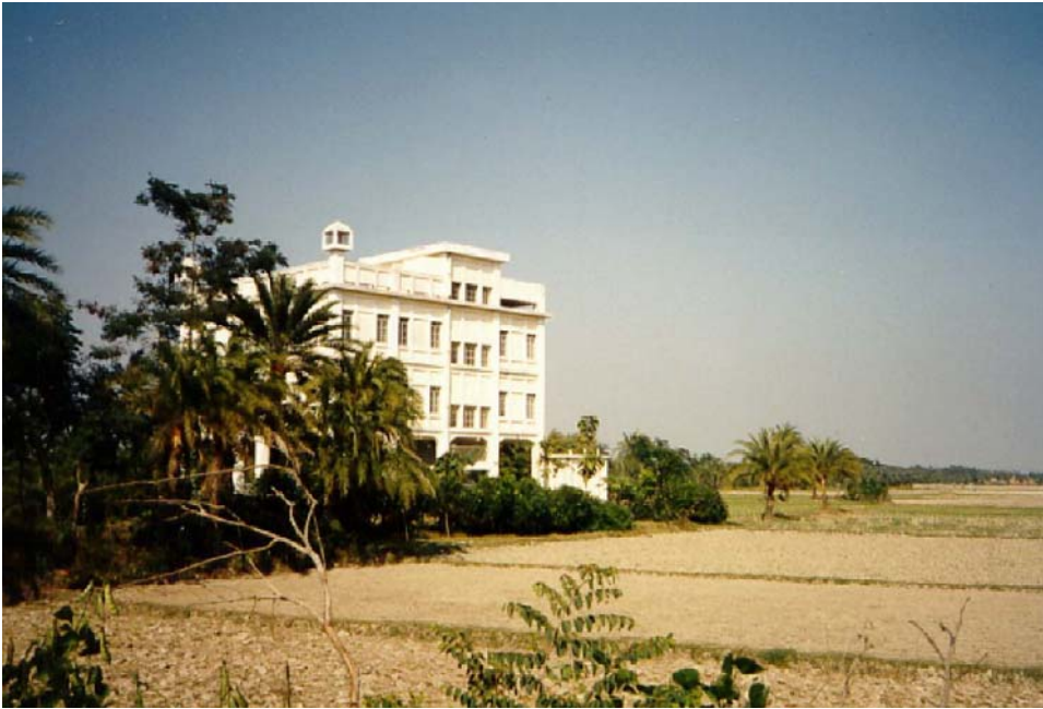
Figure 3: Cyclone shelter in Noakhali, Bangladesh
